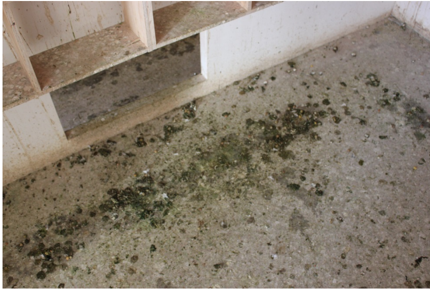
Figure 13. General appearance of loft floor (cleaned 24 hrs earlier).
